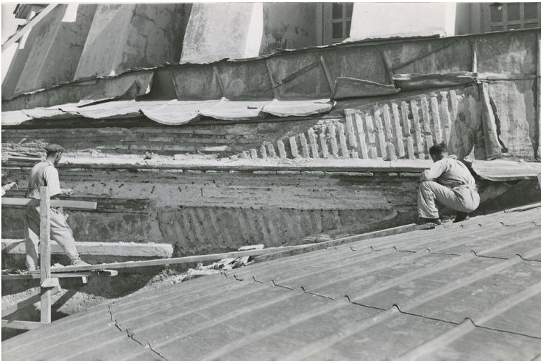
Fig. 6 – Robert Van Nice, brickwork and roofing on the main dome and a semidome, Hagia Sophia, Istanbul, Turkey ( VN-HS.00032 )
